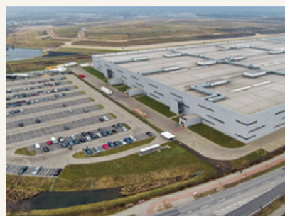
H&M logistics warehouse LOGISTICS · GERMANY
