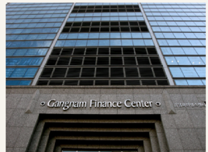
Gangnam Finance Center (GFC) PRIME OFFICE · GANGNAM, SEOUL
